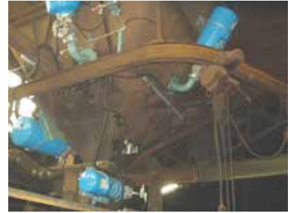
Wood chip hopper in thermal power plant
